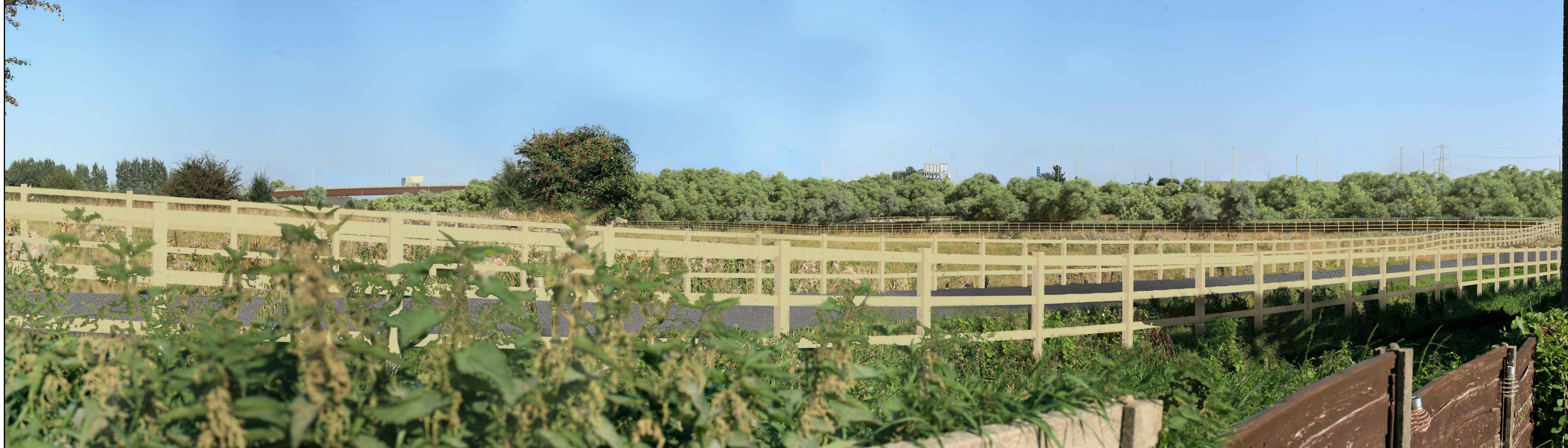
VIEWPOINT PM02: View looking east from Marston Close in Whitefield to the Simister Pike Fold Viaduct and new embankment.
